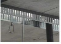
Fig. 5 ClarkDietrich BlazeFrame deflection track with factory applied intumescent tape
